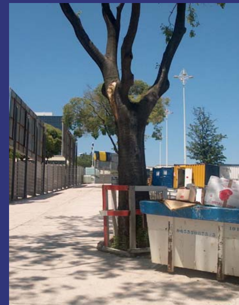
Works in Alameda
