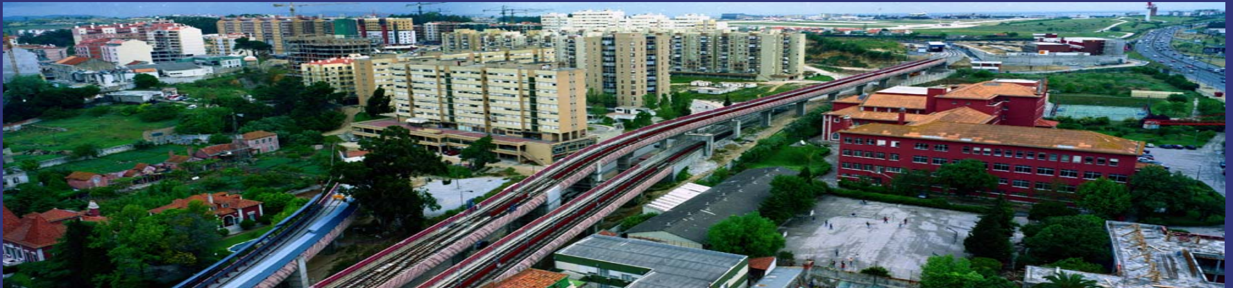
Viaduct of Campo Grande
